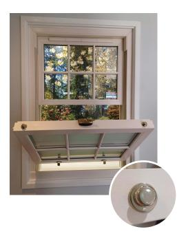
Use the lift hooks to lift the bottom sash slightly. Do not attempt to tilt the sash if it's been lifted all the way to the top.
