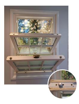
To tilt the top sash, the bottom sash must already be tilted. Pull the top sash down.
